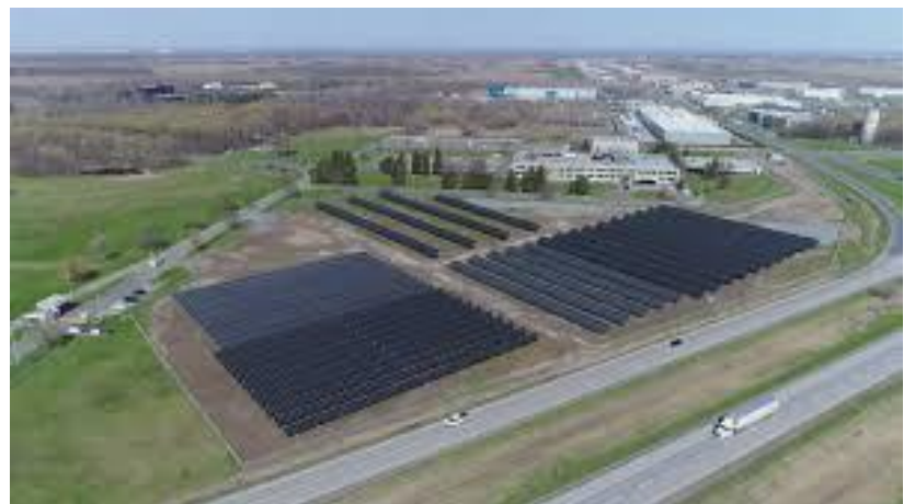
Centrale solaire Robert-A-Boyd – 2021 – Hydro-Québec
